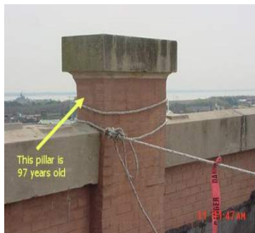
Source: OSHA Scaffolding PowerPoint Presentation
